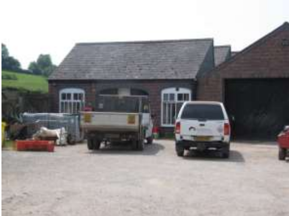
SND building at Tardebigge Basin
