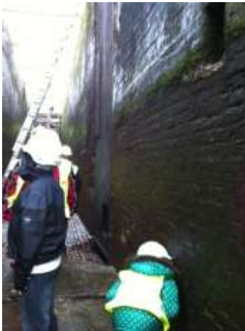
Lock 58, emptied for repairs
