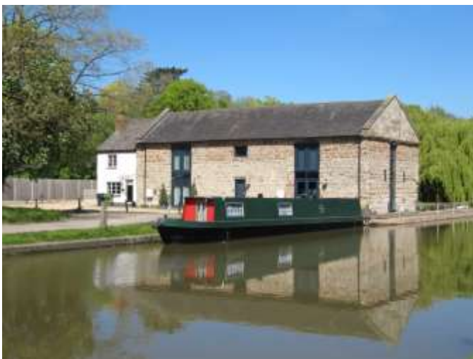
The warehouse with the cottage to the left hand side
