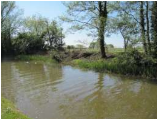
View around Locks 54 and 53 to west/north west
