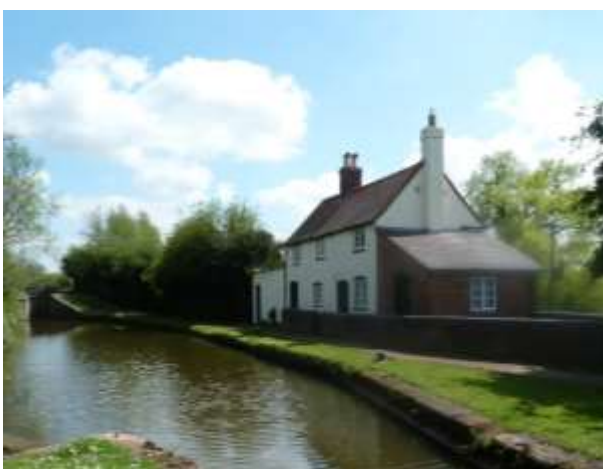
Landmark Trust lock keepers cottage
